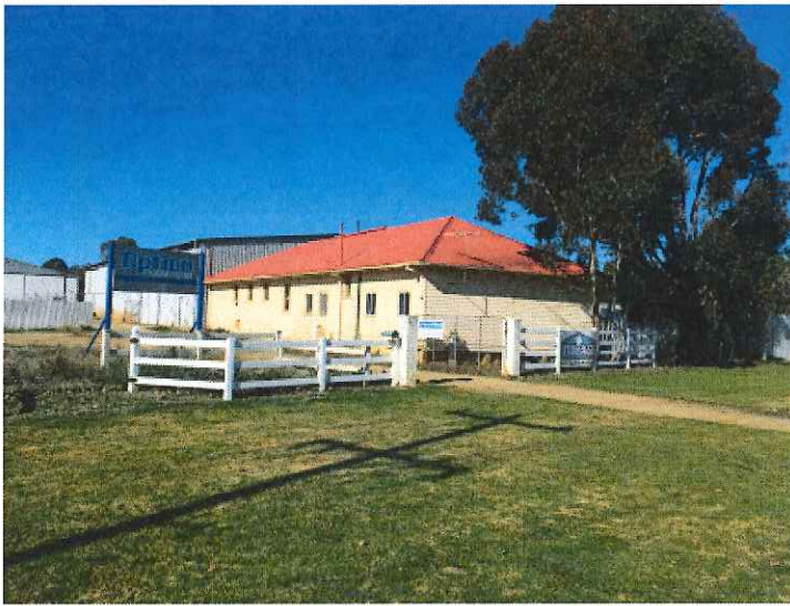
Figure 5 – Existing buildings on the northern lot addressing the Federation Avenue frontage.
